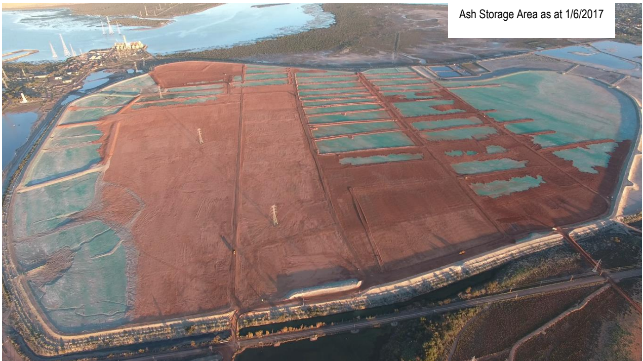
Ash Storage Area looking west.
