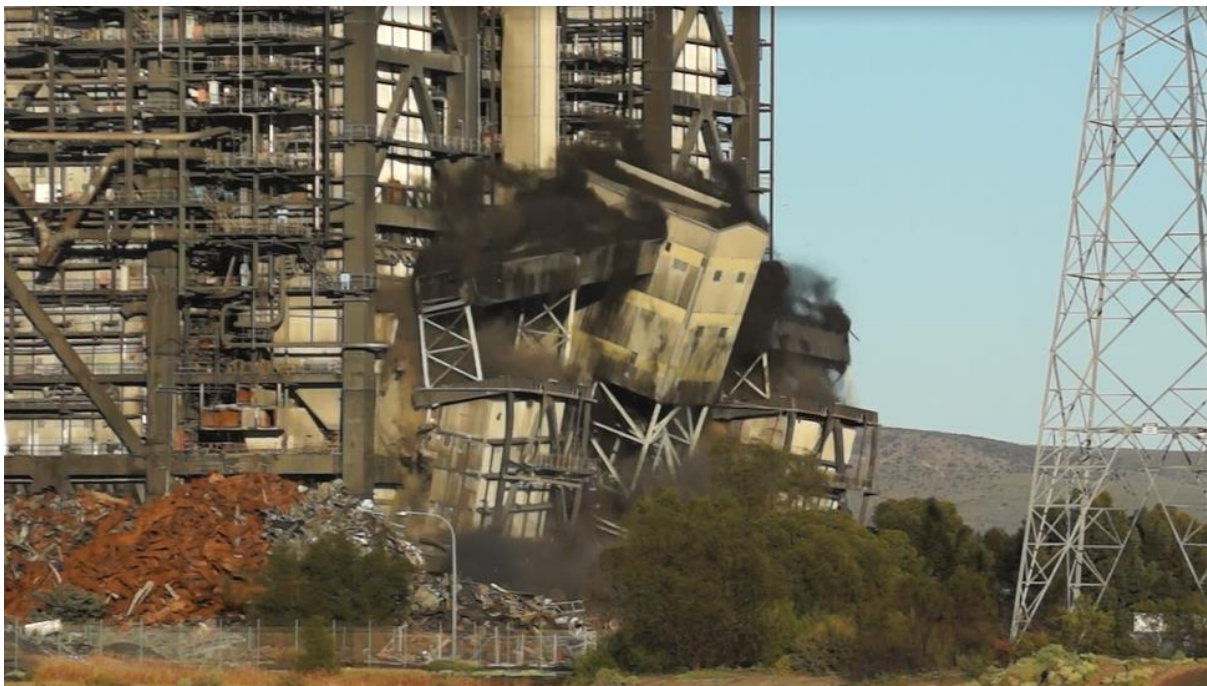
Coal Conveyor Tower G and Economiser 2 structures being felled
