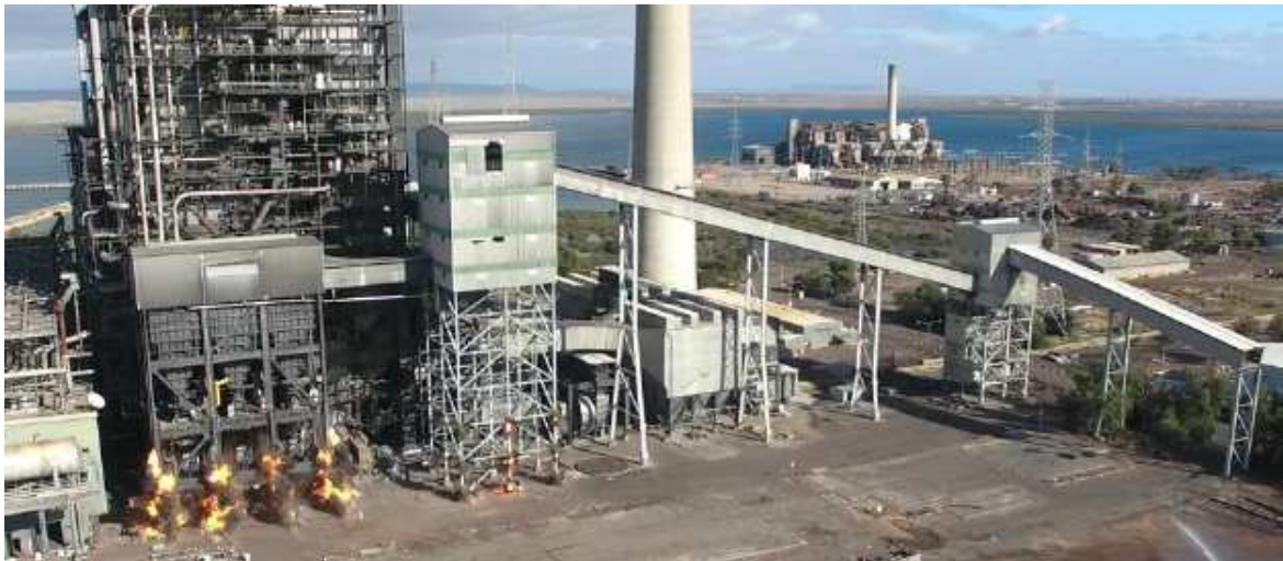
East Coal Bunker, towers and conveyor charge felling
