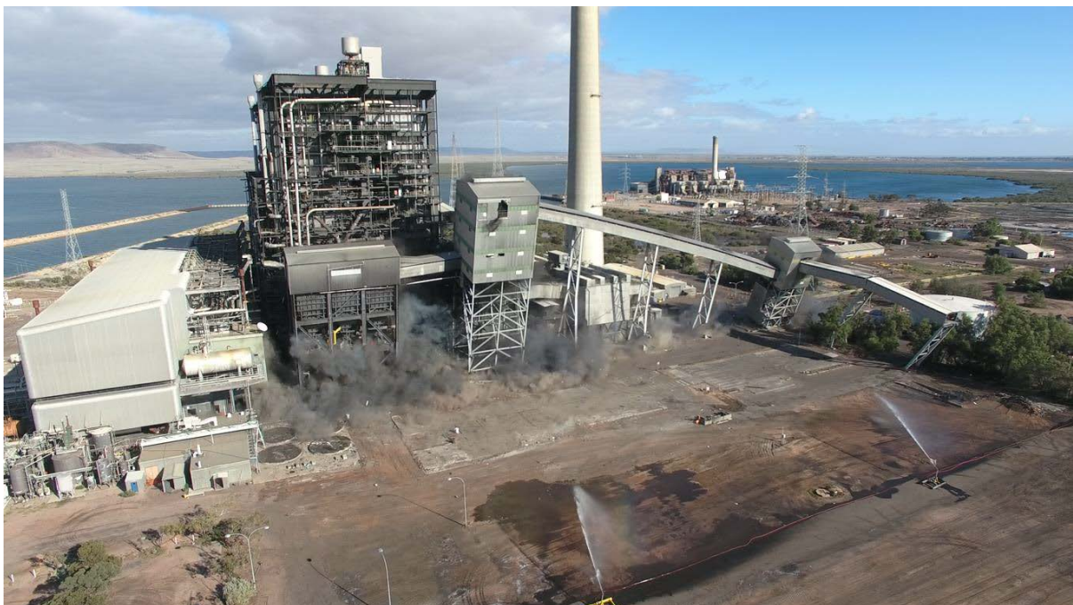
The Eastern Coal Bunker and Transfer Towers E & F being felled
