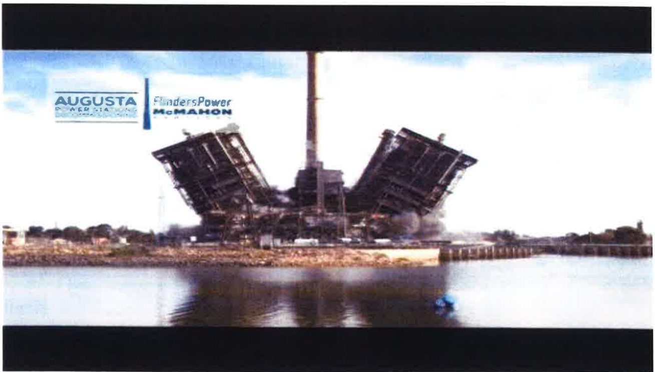
Port Augusta power station's giant boilers demolished in November 2017
