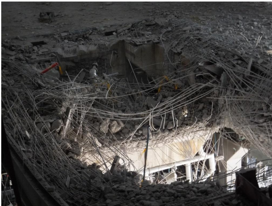
Demolished Turbine Generator Ring Beams
