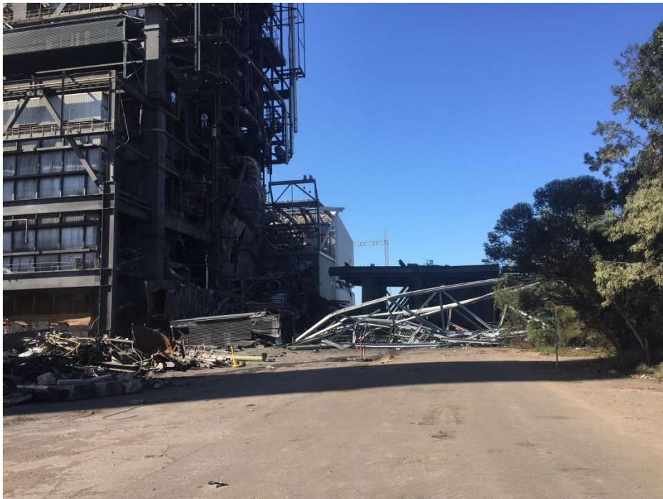
The felled Western Coal Bunker and Transfer Tower H
